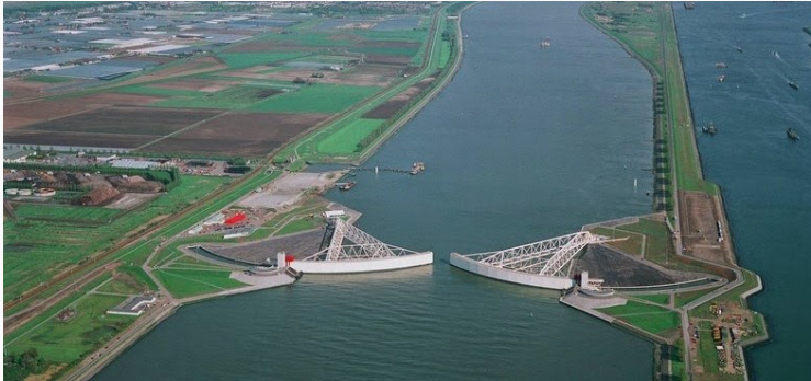
Figure 1: Maeslantkering outside of Rotterdam
