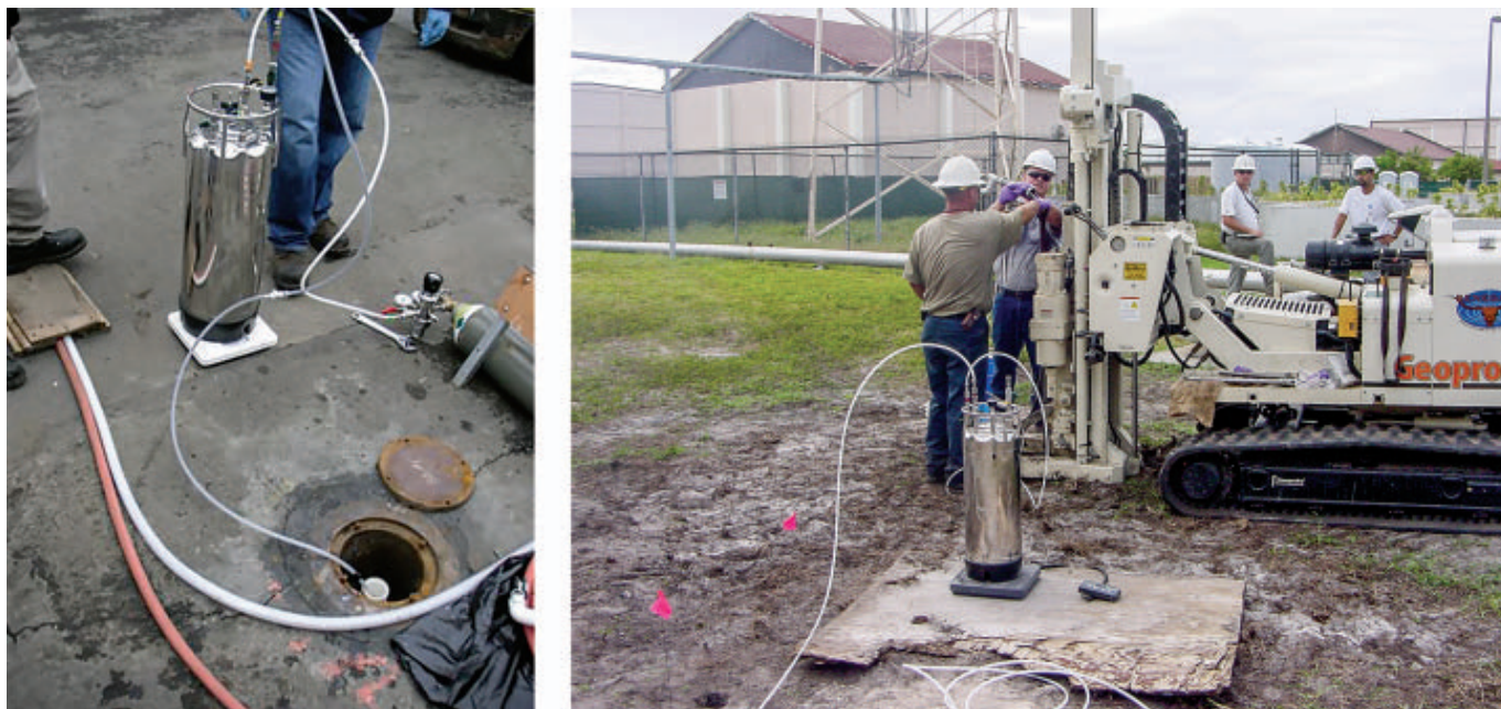
Fig. 2. Bioaugmentation with OHRB. (Left) Injection of microbial cultures containing OHRB in an injection well or (Right) direct push injection without the use of wells in aquifers contaminated with chlorinated solvents. [Reprinted by permission from Springer Nature, (22).]
